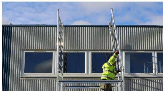
12. Add 4 rung frames ensuring the ladder is continuous. Ensure interlocks are engaged.
