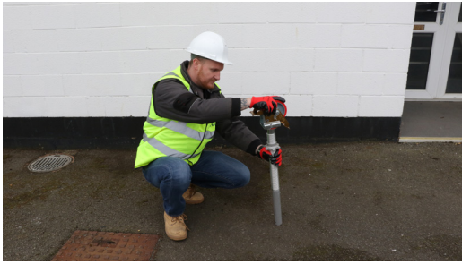
1. Insert castor wheels into adjustable legs
