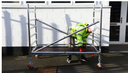
6. Fit 1 plain platform on the appropriate rung. (See base build for desired platform height). Level your tower by the adjustable legs using a spirit level as a guide.
