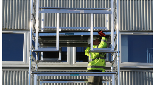
14. Fit 1 trap and 1 plain platform to the 3rd rung down. Making sure the trapdoor is with the ladder section.
