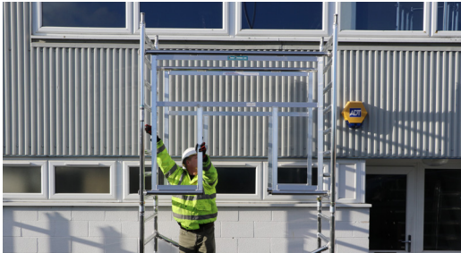
9. Fit 2 Advance Guardrail frames, hooks facing outwards ensuring the top hook is located above the top rung.
