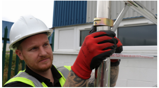
8. After adding frames, always remember to engage all your interlock clips.
