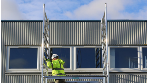
15. Continue erecting tower to final tower height repeating the AGR process (steps 12-14) as illustrated. Always ensure there is side protection to prevent falls. Platforms should be every 2m complete with handrails.
