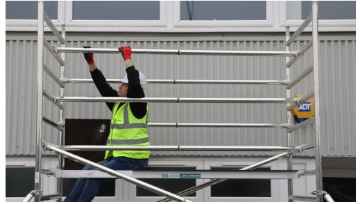
14. From a seated position, using the 3T (Through The Trap) method, fit 5 horizontal braces. 2 on the frame upright hooks facing out and 3 in the middle hooks facing down creating a secure guardrail for your access platform.
