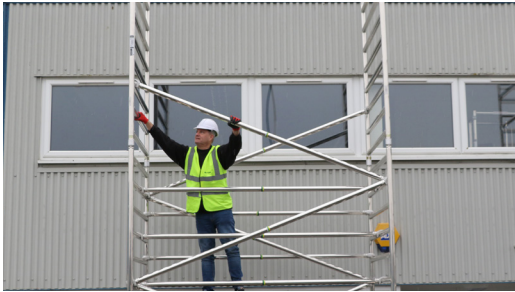
15. Continue erecting tower to final tower height repeating the 3T process as illustrated. Always ensure there is side protection to prevent falls. Platforms should be every 2m complete with handrails.
