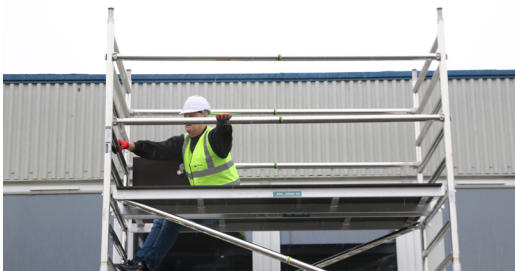
17. From a seated position using the 3T method, fit 4 horizontal braces above the appropriate rungs, hooks facing outwards.
