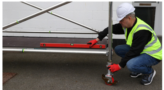
6. Fit 1 platform on the appropriate rung. (See base build for desired platform height). Level your tower by the adjustable legs using a spirit level as a guide.
