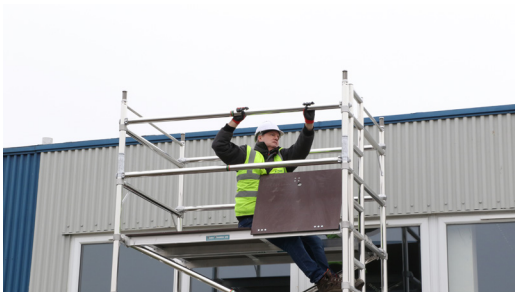
17. From a seated position using the 3T method, fit 4 horizontal braces above the appropriate rungs, hooks facing outwards.
