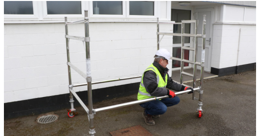
4. Fit 2 horizontal braces to the vertical member of the frames above first rung. Horizontal braces fit on from the inside of the tower facing outwards. (Integral ladder must be on the right hand side)
