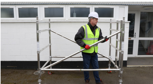
5. Fit 2 diagonal braces from the 1st rung to the 3rd rung in an alternate pattern.
