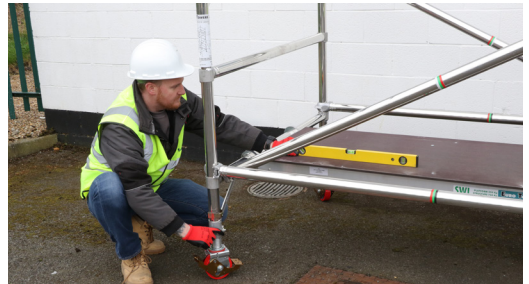
6. Fit 1 plain platform on the appropriate rung. (See base build for desired platform height). Level your tower by the adjustable legs using a spirit level as a guide.
