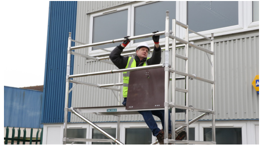
14. From a seated position, using the 3T (Through The Trap) method, fit 4 horizontal braces. 2 on the frame upright hooks facing out and 2 in the middle hooks facing down creating a secure guardrail for your access platform.
