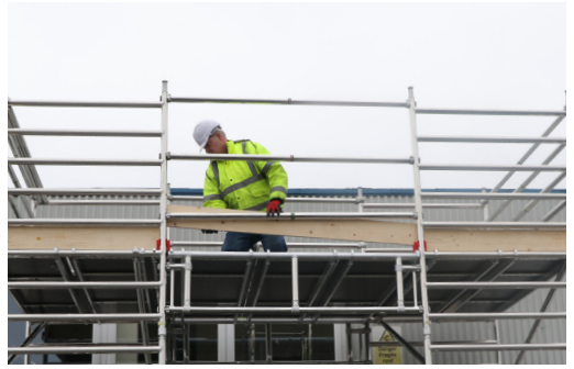
13. Fit your toe-boards to the bridge system as shown in the diagram on page 8 – ref. items 7, 8 & 9
