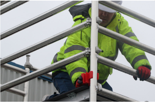
12. Add your toe-board clips to each tower upright
