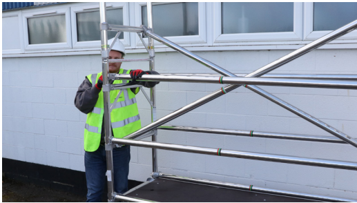
9. Fit 4 horizontal braces directly above platform to create your collective protection. Hooks facing outwards on frame uprights.
