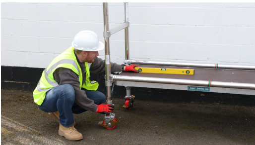
5. Fit 1 plain platform on the appropriate rung. (See base build for desired platform height). Level your tower by the adjustable legs using a spirit level as a guide.
