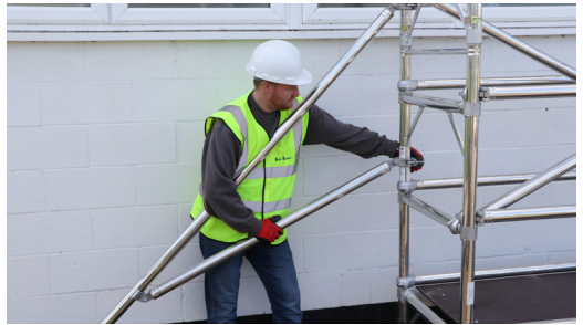
10. Fit 4 stabilisers at earliest opportunity keeping lower arm as horizontal as possible.
