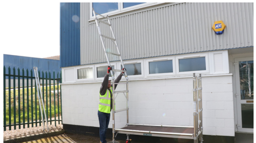
6. Add further frames ensuring the ladder is continuous.
