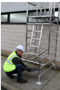
Fit the step platform at the base of the unit as shown.
