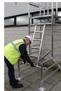
Fit the ladder 1 rung below the working platform. Pivot the rung until the hook is facing downwards and clip into place.
