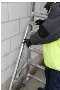
Fit stabilizers on both sides of the unit.
